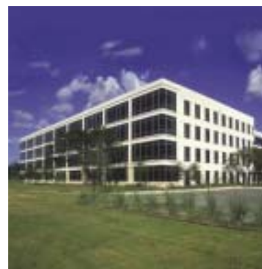
Austin Research Park - Buildings III & IV Austin, TX
